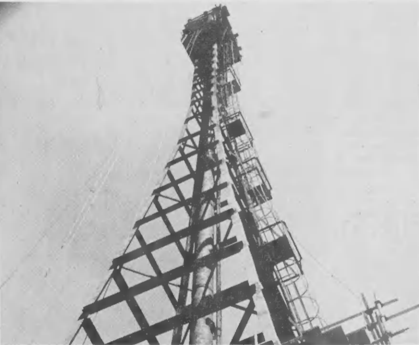
HIGH UP, about 280 feet up, scaffolding encases the top of the Alky flare. The scaffolding presents an interesting, and peculiar, shape to the top of the slender unit. The aerial below shows Lago's main ingress. HOPI HALTO, como 280 pia halto, stelashi ta encerra e top di e chimenea di Alky Plant cu ta manda vlam. E estructura aki, cu a worde instalá no mucho tempo pasá pa trabao di mantencion, ta presenta un figura interesante y raro na e top di e chimenea delegá.
